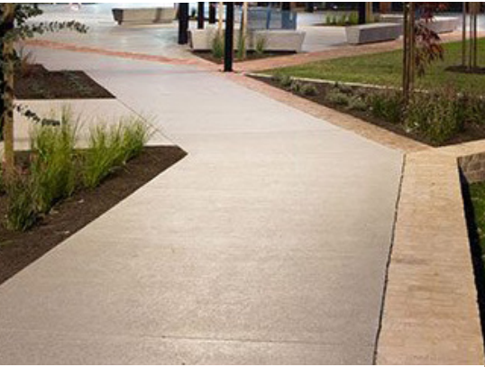
P2: Pavement Type 2 - Insitu exposed aggregate concrete
