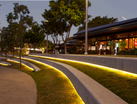
W2: Wall Type 2 - Insitu concrete amphitheatre walls
