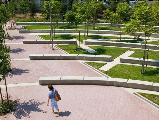
W1: Wall Type 1 - Insitu concrete seating walls
